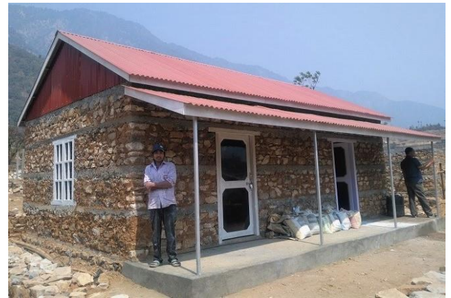
Figure 2: House owner Som Bahadur Ghalng Makwanpur Gadhi Rural Municipality-08. He has been working in reconstruction for 3years as a mason. He received second tranche and verified for third tranche by NRA field base engineer. His house looks attractive and also earthquake resistant like as all horizontal, vertical element provided also light material used. His house is two rooms with one story and total cost of this house is 6lakhs.
