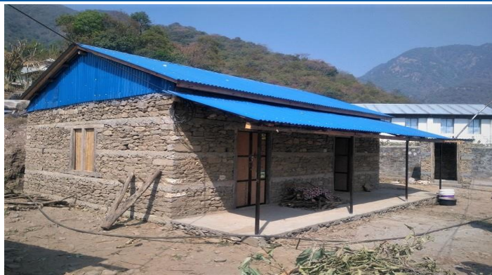
Figure 3: Stone in mud mortar with RCC band, flexible roof and all Horizontal & vertical element provided. House owner received second tranche and verified for third tranche by government engineer. Location of this house is Makwanpur Gadhi-o8 and total cost of this house is around 6lakhs.
