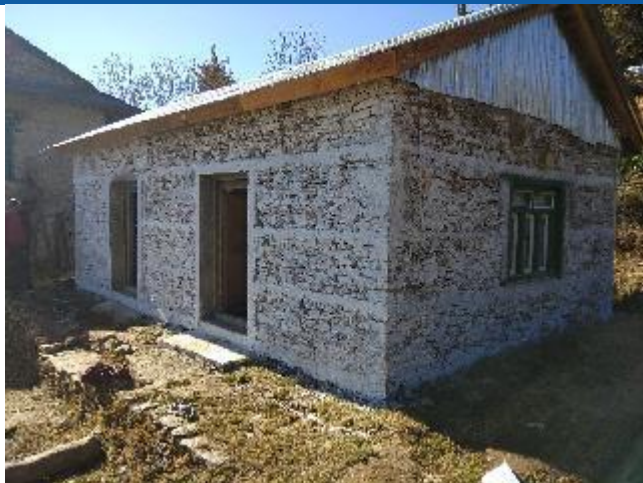
Caption: The house of Ang Chongba Sherpa constructed in Preeti of Umakunda Rural Municipality (4). The house owner has received the second tranche of reconstruction grant.
