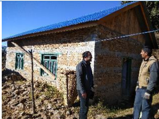
Caption: The constructed house of Nima Sherpa being observed by DLPIU Sub Engineer and M&E Consultant. The house owner has received second tranche of reconstruction grant.
