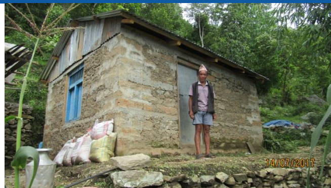
Caption: Kalika Rural Municipality ward no 5, Rasuwa House Owner Name: Bir Badhur Bulun, Construction completed, stone masonry, received 3rd tranche.
