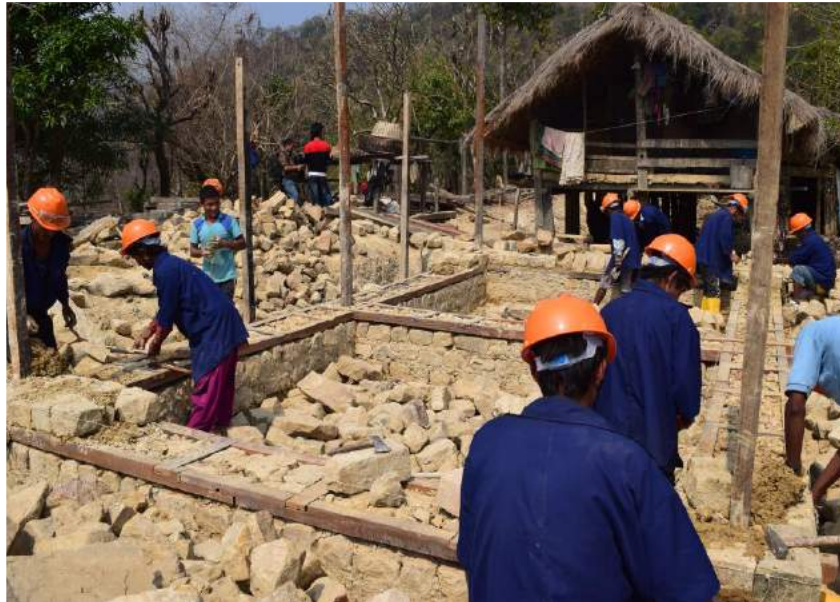
Kapilakot-5, Sindhuli, Stone Masonry with Mud Mortar, Bands provided
