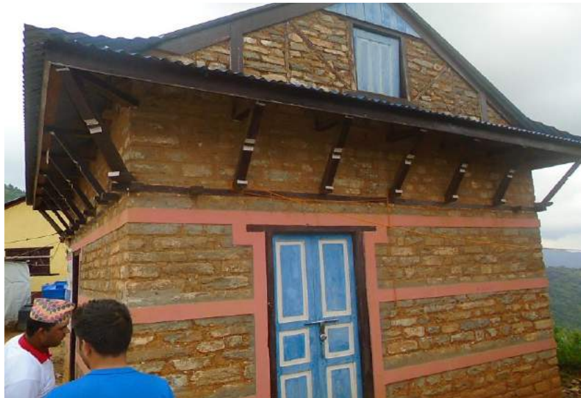
Rampur-7, Single Room House, proper band provided, Nepal Red Cross Society, Model House
