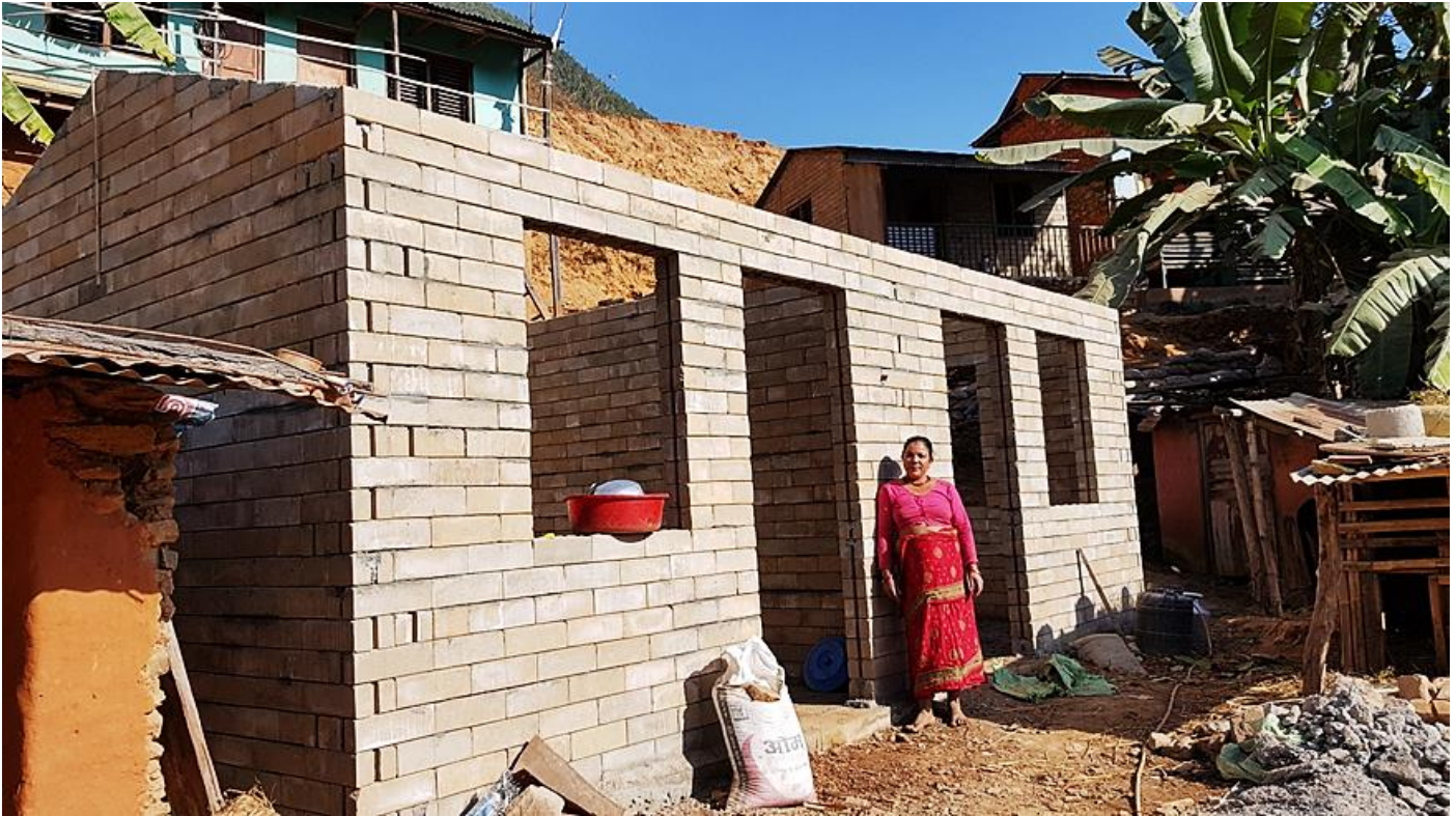
Bidur-6, Nuwakot: Shanta Sunar has constructed her home using Compressed Stabilised Earth Blocks (CSEB) but has not received the second tranche and so her reconstruction has stalled.
