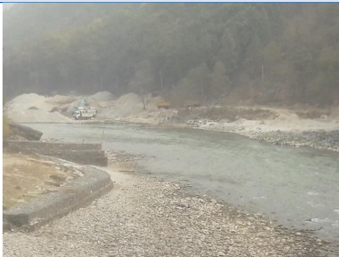
Caption: Extraction of river bed material in Tamakoshi River by a crusher plant. Extraction is high with the increased demand of construction material.
