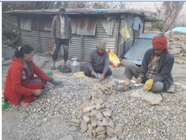
Caption: House owner and his neighbor friend is busy in crushing of stone into small pieces to meet the gravel requirement for concreting.
