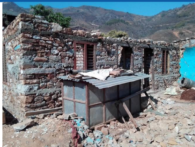
Name:- Bholu Bhandari Address: - Kumpur, Siddhalekh Rural Municipality Type of house:-Stone Masonry in Mud Mortar Get 2 nd Tranche
