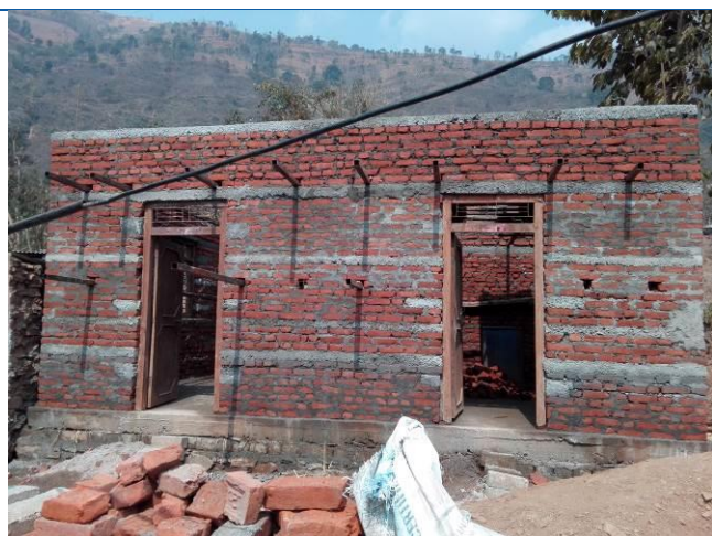
Name :- Chandra Kumari Newar Address: - Kumpur, Siddhalekh Rural Municipality Type of house:-Brick Masonry in Cement Mortar. Approved for 2 nd Tranche.
