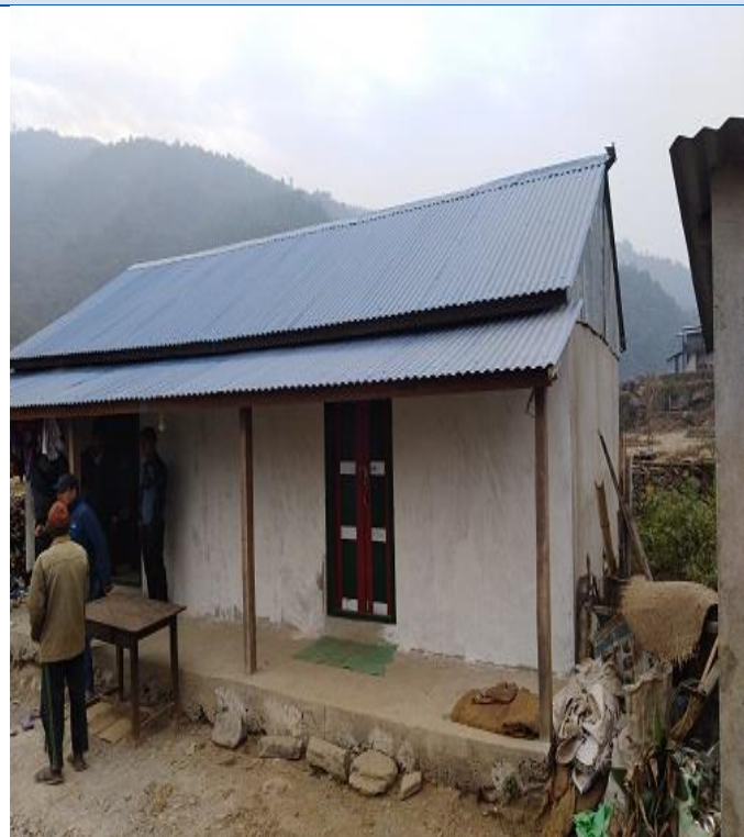
Caption: Massonary structure building built by HELVETAS in Bastipur ward no-02 of Ghanglake Rural Municipality of Sindhuli district. Construction of this house is completed and beneficiary had got government 3 rd tranche.
