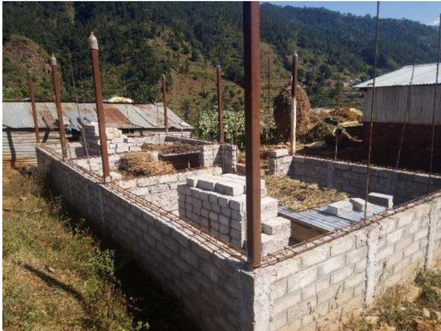
*Bhimtar, Indrawati Gaupalika, Sindhupalchok: the house is being constructed using hollow concrete blocks with vertical steel posts of 75mm x 75mm. The house has not yet been approved for the second tranche as it is still under review.*
