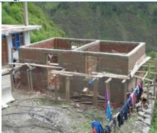
Brick masonry with cement at Parbatikunda Rural Municipality ward no 4 (Gatlang). Received 2nd tranche. House owner name Tara Tamang
