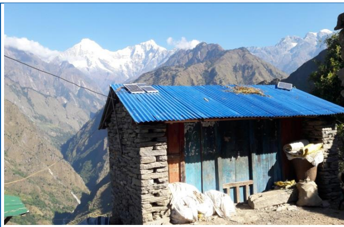
Address: - Sertung, RubiValley Rural Muicipality Type of house: - load bearing structure using dry stone with CGI sheet roofing.
