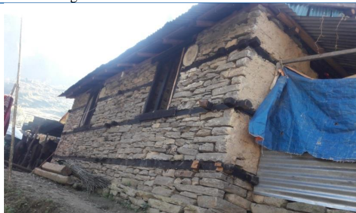
Address: - Sertung, RubiValley Rural Muicipality Type of house: - load bearing structure using dry stone with slate roofing.
