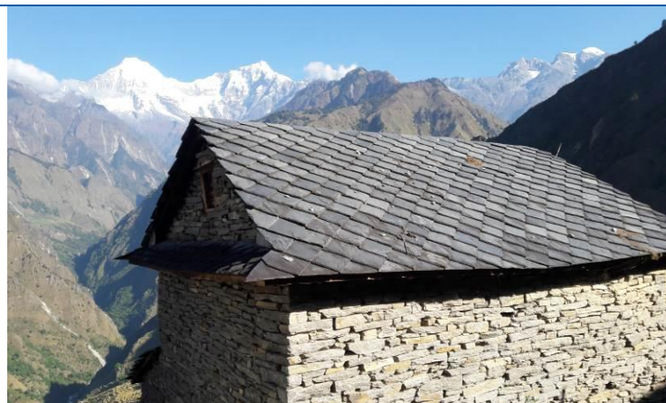
Address: - Sertung, RubiValley Rural Muicipality Type of house: - load bearing structure using dry stone with slate roofing.
