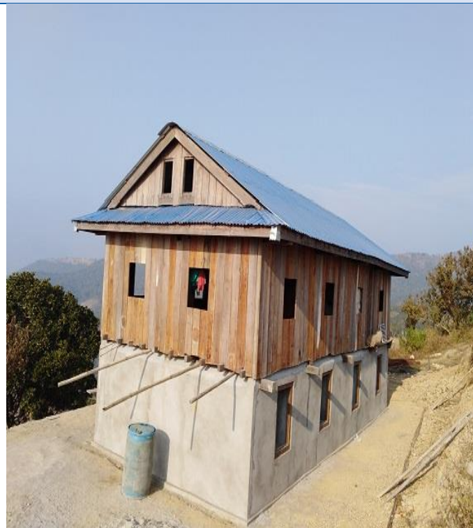
Caption: Hybrid Structure building of Marin Gaunpalika ward no- 02 of Sindhuli district. Construction of this house is completed and the beneficiary is waiting for 3 rd tranche.
