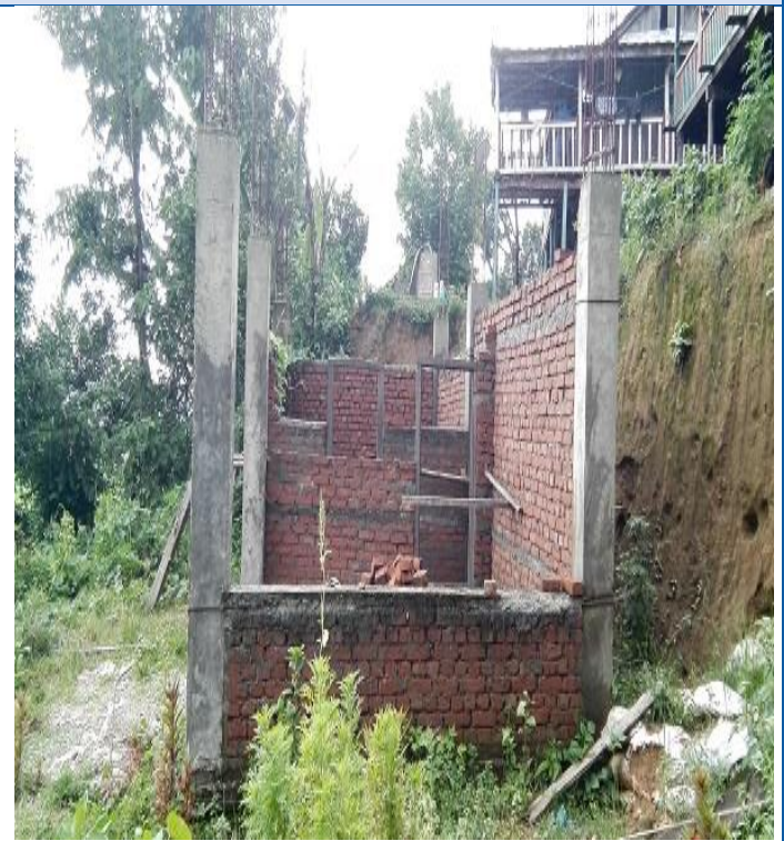
Caption: RCC frame structure building of Marin Gaunpalika ward no – 05 of Sindhuli district.
