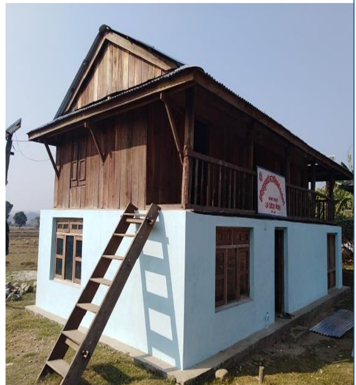
Caption: Hybrid Structure building of Hariharpurgadhi Gaunpalika ward no- 02 of Sindhuli district. Gaunpalika office is in this building, construction of this house is completed and the beneficiary is waiting for 3 rd tranche.
