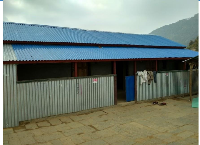
Caption: Mucchok ward no. 5, Ajirkot Gaupalika, Gorkha district, finished brick masonry cement mortar house of M/s Anita Gurung, which has been approved for third tranche by DUDBC and forwarded by DCC to the bank
