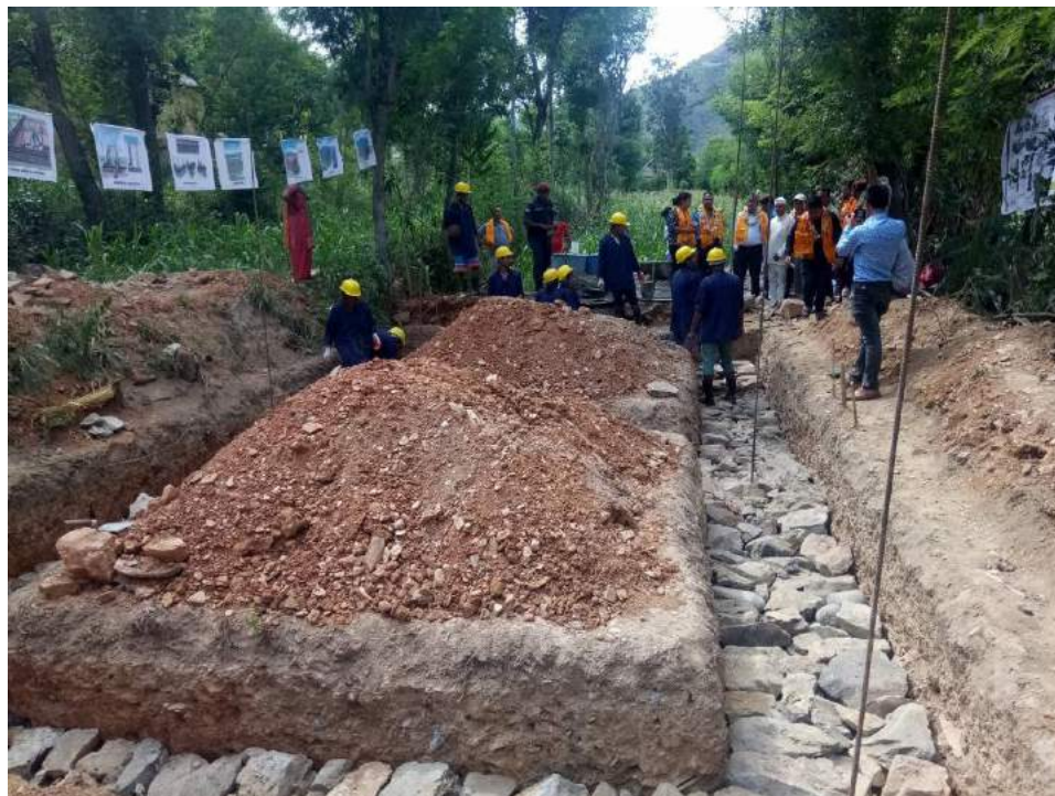
Masons training in Sunkoshi Rural Municipality, Sindhuli
