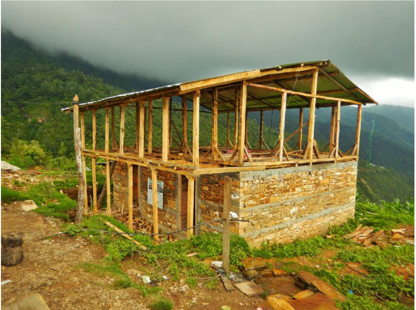
Hybrid structure, Baideshwor Rural Municipality-4, Dolakha
