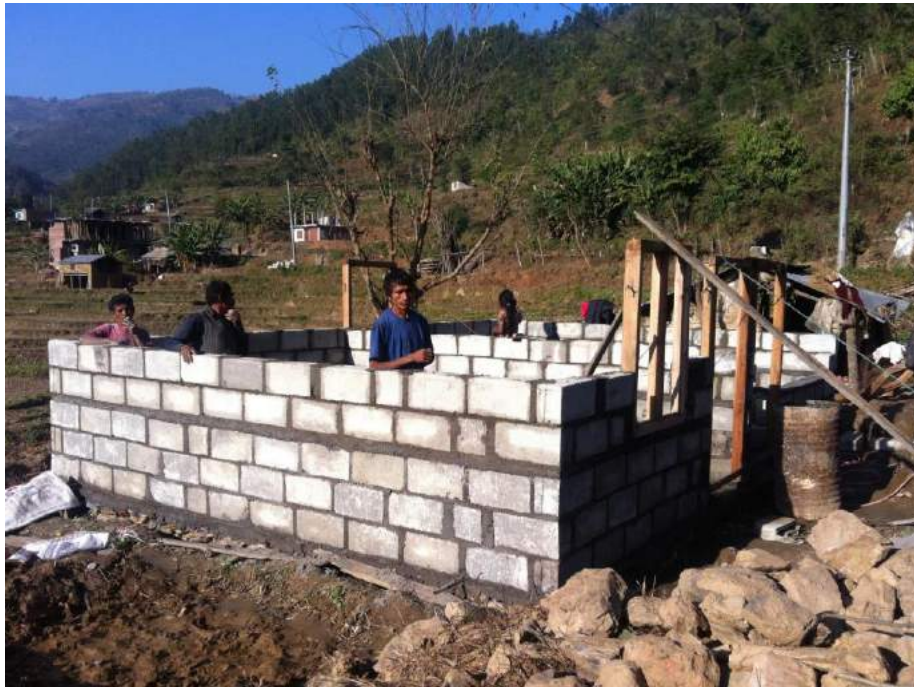
Hollow concrete block house construction in Dhading
