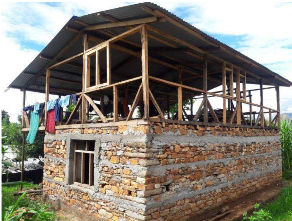
Hybrid structure, Baideshwor Rural Municipality, Ward No. 6
