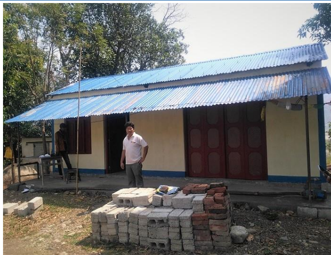
Figure 2: Raksirang Rural Municipality-05, house owner Thaku Ram Thing. He has been received all government tranches. The typology is Brick in cement mortar with flexible roof, two rooms with one story. The construction cost is around 5.5lakh.
