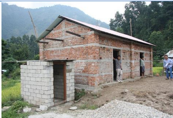
Figure 2: Brick in cement mortar, two rooms with RCC band, flexible roof. Sun Maya Tamang, Kailash rural municipality-10. She received all government tranches of housing grant.
