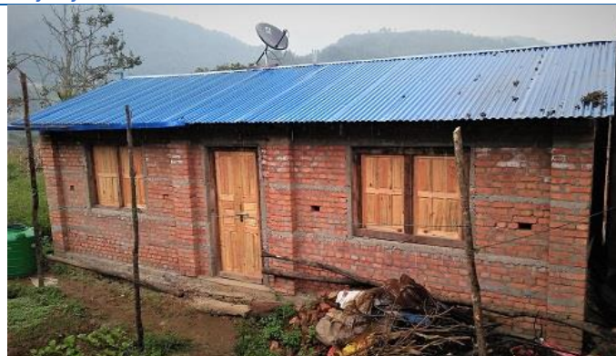
Figure 6: Thaha Municipality-10, brick in cement mortar with RCC band, two rooms with flexible roof. The total construction cost is around 7.5lakh.
