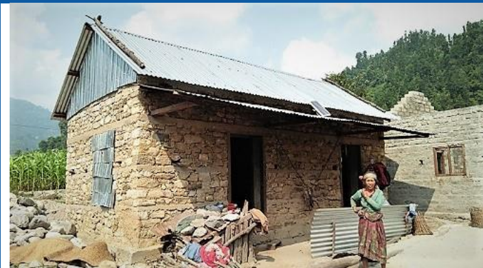
Figure 3: stone in mud mortar with RCC band, two room and flexible roof with light gable material. Chepang community, House owner: Goma Praja, Kailash Rural Municipality-03. She received all government grants. The tentative construction cost is around 3.5 lakh excluding their contribution.
