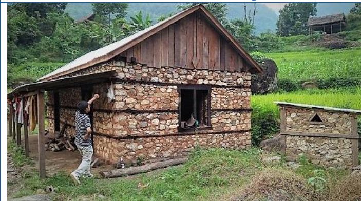
Figure 5: Stone in mud mortar with wooden band. Provided all vertical post, flexible roof and two rooms. This house is eligible for third tranche. House owner: Durga Thing, Kailash-03. She received 2 nd tranche and verified for 3 rd tranche.
