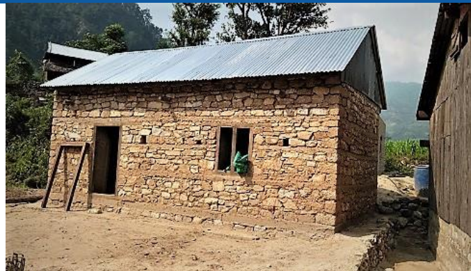
Figure 4: stone in mud mortar with RCC band, two room and flexible roof with light gable material. Chepang community, House owner: Bhim Bar Praja, Kailash Rural Municipality-03. He received second tranche and verified for third tranche.
