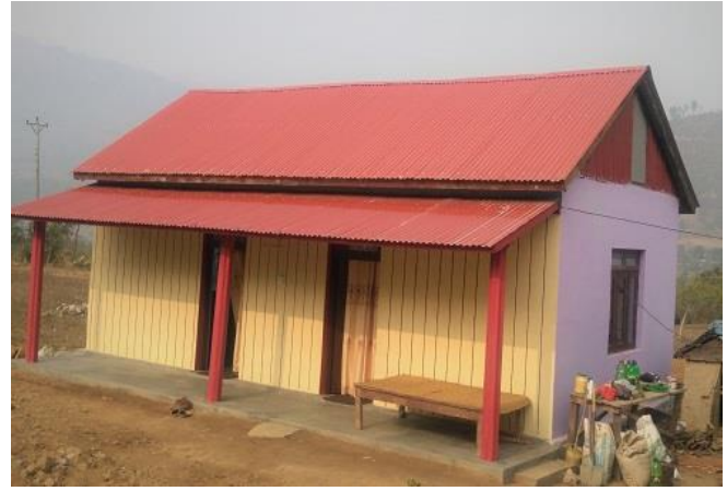
Figure 2: Raksirang Rural Municipality, Makwanpur. House owner Anita Shah made up brick in cement mortar with flexible roof. Totally earthquake resistant building with two rooms, one story & an attic. House owner has received 2 nd tranche and processing for 3 rd . The house is completed and grand total cost of building is 6 lakhs.
