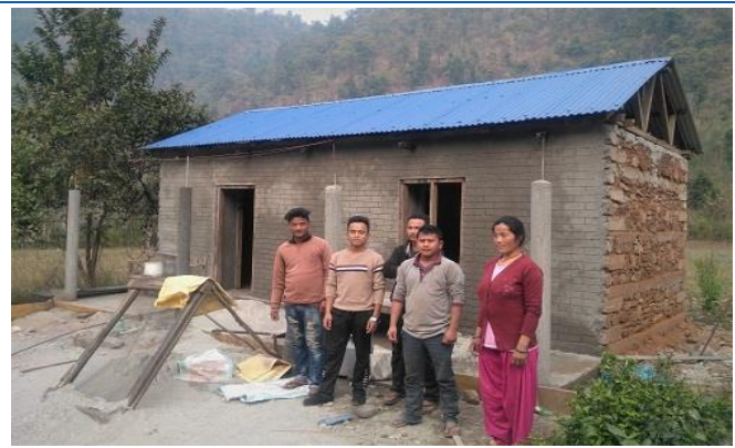
Figure 4: Stone in mud mortar with flexible roof, one story with RCC band. House owner: Dal Bahadur Syantan, this house verified for second and third tranche. Tentative cost of this building is 4.5lakhs excluding their jointly working labor cost. Location is Raksirang RM-03.
