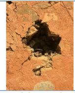
These hole ares provided to insert dowel bar for connecting column and wall.
