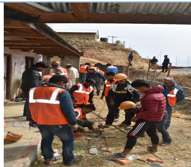
Practical in mason training in Sindhukot.
