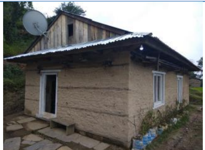
Caption: The house of Sujit Bishwakarma of Rawadolu VDC. The owner has received the second tranche of reconstruction grant. The house has been completed and has been processed for third tranche of reconstruction grant.
