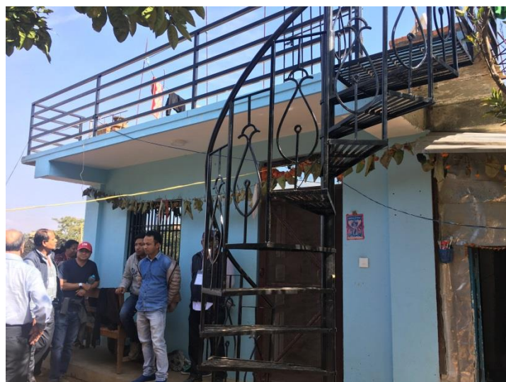
Chapagaun Ward no. 10, 3 rooms Load bearing structure with RC roofing. The house in completed with the material support worth 300,000 NRs and remaining from the beneficiary.
