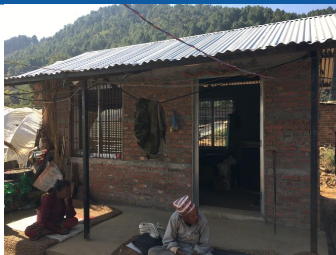
Chapagaun Ward no. 10, single room single storey load bearing structure with CGI roofing.
