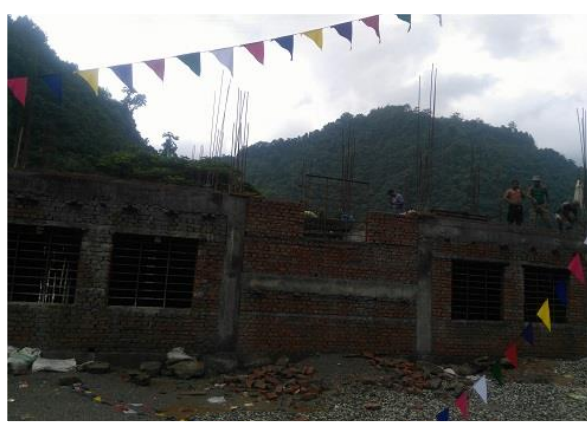
School building underconstruction at Bhaise VDC current Bhimfedi Rural Municipality-1 Makwanpur.
