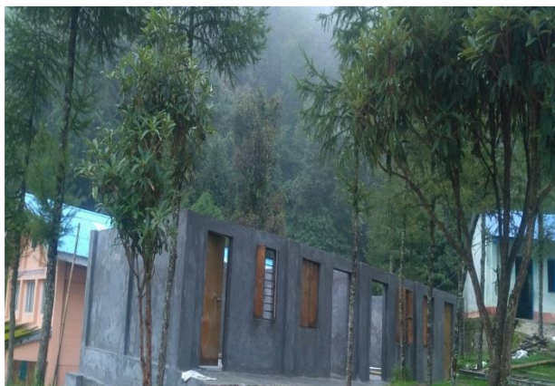
School building underconstruction (Lakali Basifaat MA BI Namtar Makwanpur) .
