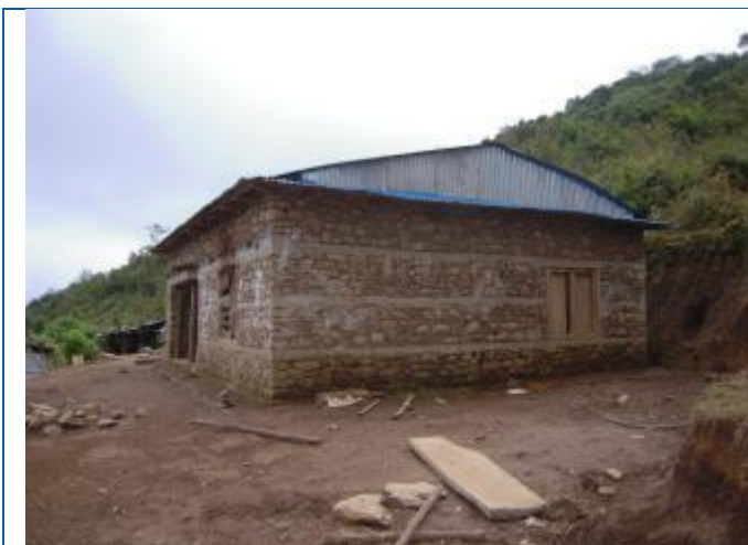
Caption: The house of Devi Dhoj Karki constructed in Saipu, Likhu Tamakoshi Rural Municipality-2. The owner has received second tranche of reconstruction grant and has been forwarded for third tranche.
