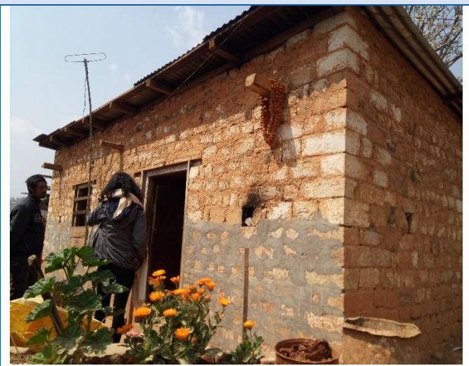
Devasthan, Ward No. 8, Chaimale, Dakshinkali Municipality, Stone Mud Masonry house with CGI roof. The house owner was recommended to follow up with engineers at Dakshinkali Municipality for undertaking retrofitting of the house in order to receive 2 nd tranche.
