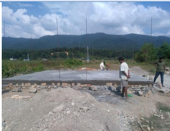
Figure 2: Under construction house and processing for second tranche at Manhari Gaupalika.
