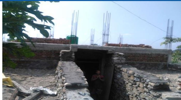
Caption: RCC frame structure with brick masonry at Manhari 01 current Manhari Gaupalika 06, owner: Sarita Sherstha. She received second tranche and processing for third tranche.
