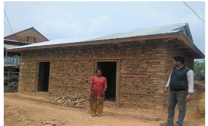
Figure 3: Indrasarowar Rural Municipality-01, house owner Nar Bahadur Bist. Stone in mud mortar with timber band and flexible roof. He has received all tranches of government grant. The tentative construction cost of this building is 5lakh..
