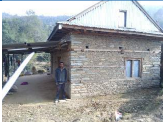
Caption: The constructed house of Chamar Singh Tamang, resident of ward number 7, Khadadevi, of Khadadevi Rural Municipality. The house is constructed using stone in cement mortar. The RC bands have been provided to the house. He has received third tranche of reconstruction grant on 24 th Poush 2074. The house was completed in 6 lakhs
