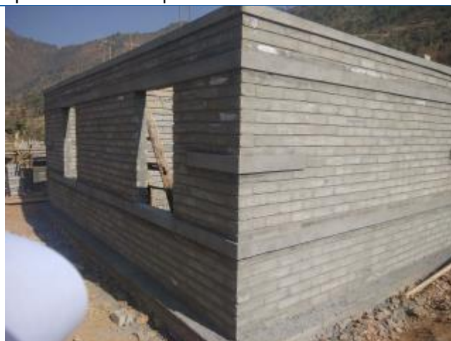
Caption: The two room structure of tranche Ram Bahadur Shrestha, resident of Bhirpani, Khadadevi Rural Municipality-3 being constructed by using CSEB interlocking bricks. The blocks are produced by vendor in Mulot and have been constructing the earthquake resilient house at 6.5 Lakhs. The house has been recommended for second tranche on Mangsir 2074 but has not received the tranche yet.
