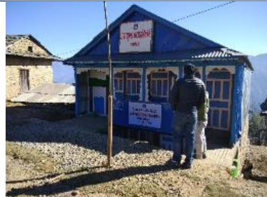
Caption: The premises of Umakunda Rural Municipality where the office for the chairperson, vice chairperson, and technical staffs is situated.
