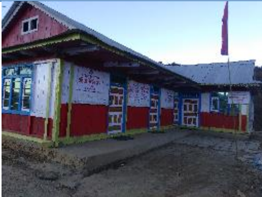
Caption: The service centre of Umakunda Rural Municipality where the department of women and children development, livestock, health and agriculture related services are provided.
