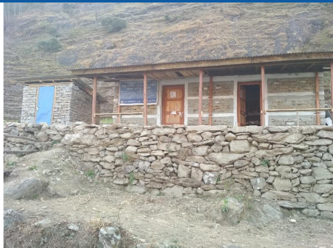
Caption: Dongchet ward no. 1, Manbu, Aarughat Gaupalika, Gorkha district, demo house constructed by SSICDC/CRS which has been handed over to Tyeghar Community Forest Users Committee
