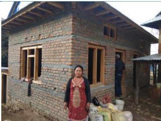
Caption: The house of Bhakta Laxmi Thapa Magar of Dimipokhari of Sunapati Rural municipality-2. The house has been constructed using brick in cement mortar. The house consists of two rooms. The owner has not received all three tranches of reconstruction grant.
