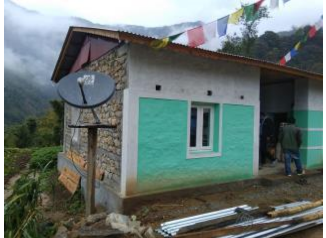
Caption: The house of Kale Tamang of Doramba of Doramba Rural municipality. The house has been constructed using stone in mud mortar. RC band has been provided to the house. The house consists of three rooms. The owner has received second tranche of reconstruction grant and have been forwarded for third tranche.
