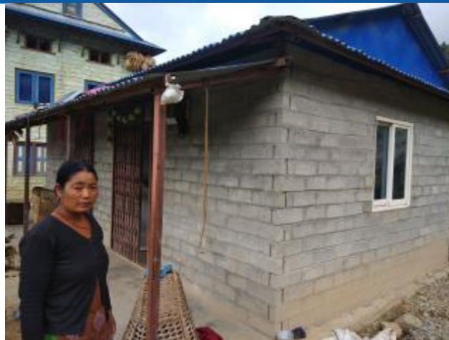
Caption: The house of Amrita Thapa Magar of Dimipokhari, Sunapati Rural Municipality-2 being constructed. The house has been constructed using interlocking blocks. The house has two rooms. The owner has received second tranche of reconstruction grant. The house has been constructed in 5 lakhs.
