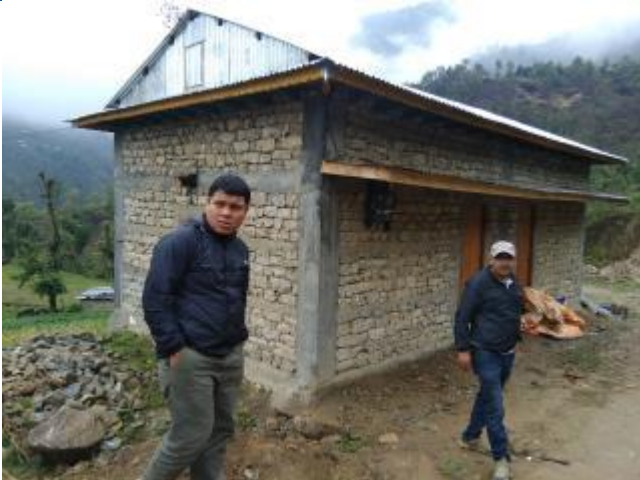
Caption: The house of Salam Tamang of Doramba of Doramba Rural municipality. The house has been constructed using stone in mud mortar. RC band has been provided to the house. The house consists of two rooms. Columns have been provided to the building at the corner. The owner has received second tranche of reconstruction grant.
