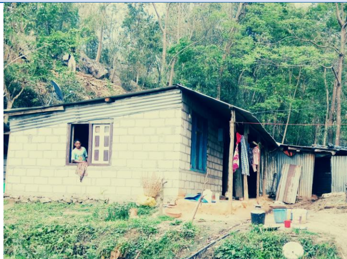
Sisneri, Ward No. 9, Lamatar, Mahalaxmi Municipality, Blocks made house. The house owner has approved building drawing. The 2 nd tranche is in pending stage.
