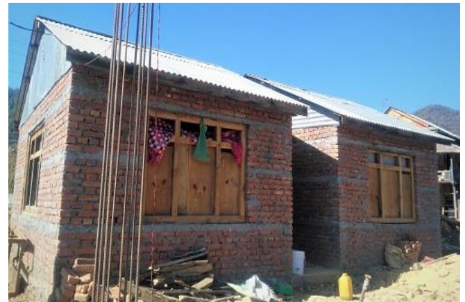
Figure 2: Earthquake resistant buildings with one room, one story an attic at IndrdaSarowar RM-5. House owner Sanu Kari and Shiv Bahadur Karki, they completed the house & process in second and third tranche.
