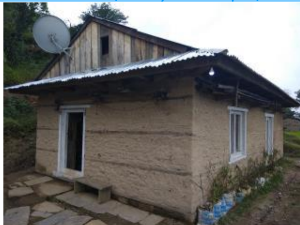
Rawadolu VDC, Okhaldhunga. House owner Sujit Bishwakarma, has received the second tranche of reconstruction grant. The house has been completed and has been processed for third tranche of reconstruction grant.
