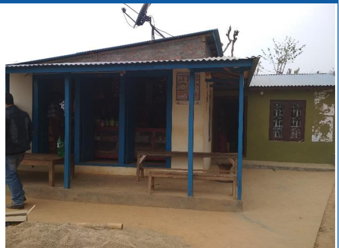
Caption: Jyamiswara – 6, Ghairung of Sahid Lakhani Rural Municipality, completed brick and cement mortar house with RCC band and wood and frame. House owner is Ms. Lina Thapa, who is also a trained mason. She has already received all tranche.
