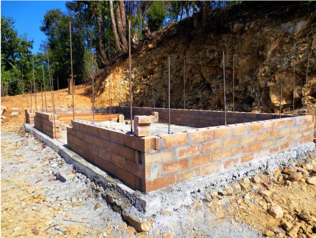
Demonstration house, using locally produced earth bricks, under construction in Kot Dada, Godawari Municipality through collaboration between Build Up Nepal, Build Change, and We Help Nepal.
